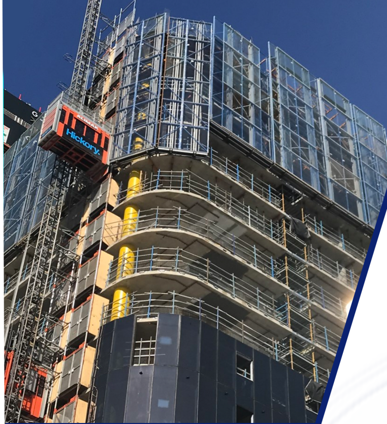
Construction site use
