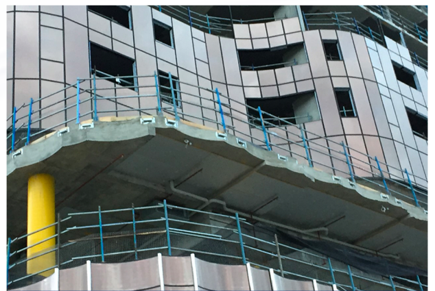
Construction site use
