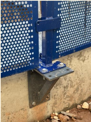
Bolt on side wall
