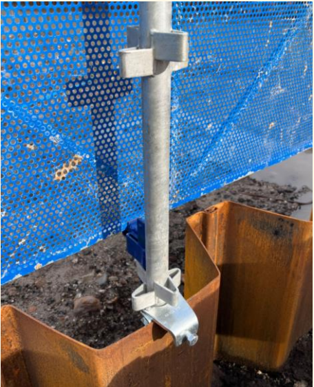
Clamp on sheet pile
